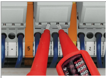
Easy testing at touchproof contacts
