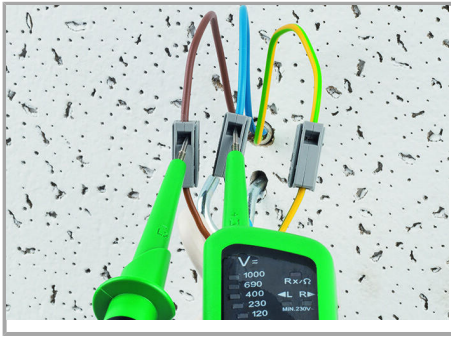
Testing via separate test ports.
