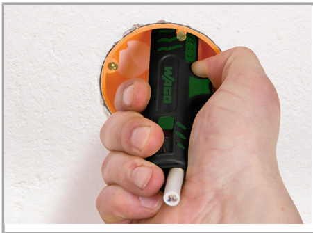
Stripping a cable sheath.
